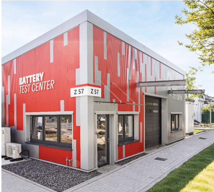
Henkel's Battery Test Center, an integral part of its groundbreaking Battery Engineering Center.
