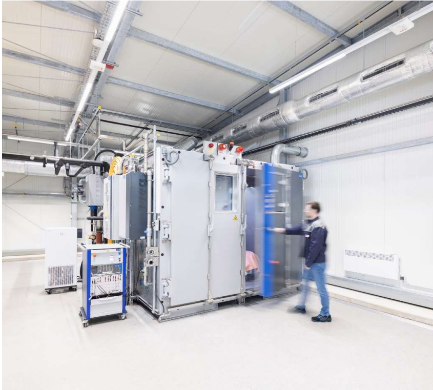
Inside the Battery Test Center, where a wide range of temperature and humidity tests are performed on active batteries through the climate chamber.
