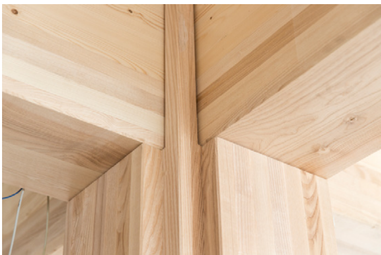
Close up of a joint and seam of wood panels.
