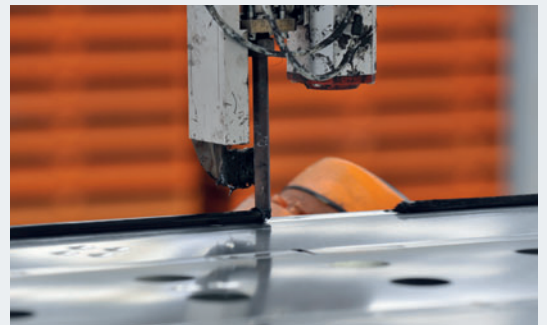
The Terostat MS adhesive is extruded automatically onto the steel frames to which the mirrors are then bonded.
