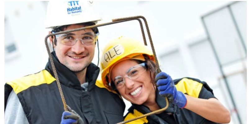
Together with the organization Habitat for Humanity, teams from Henkel’s Adhesives for Consumers, Craftsmen and Building business area supported the construction of an apartment building for families in Veles, Macedonia, in 2017.
