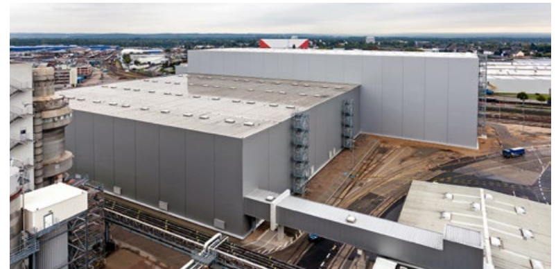
In 2017, we expanded our fully automated high-bay warehouse at our headquarters in Düsseldorf, Germany. The warehouse can now hold about 53 million packs of laundry detergent and cleaning products on a floor space of 24,000 square meters. In line with the wall-to-wall concept, the high-bay warehouse is directly connected to the Laundry & Home Care production facility, which cuts transport requirements.
