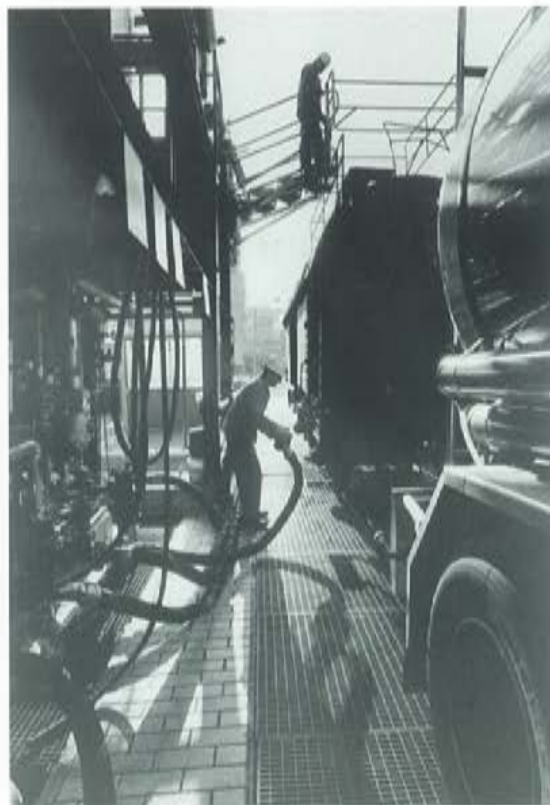
A collector zone ensures that no chemicals escape into the soil due to sudden, unexpected leakage when tank trucks are being discharged.
