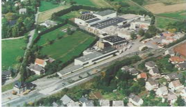
Preventive measure by Henkel Oberflächentechnik in Herborn-Schönbach: An automatic measuring station monitors the rainwater drain.
